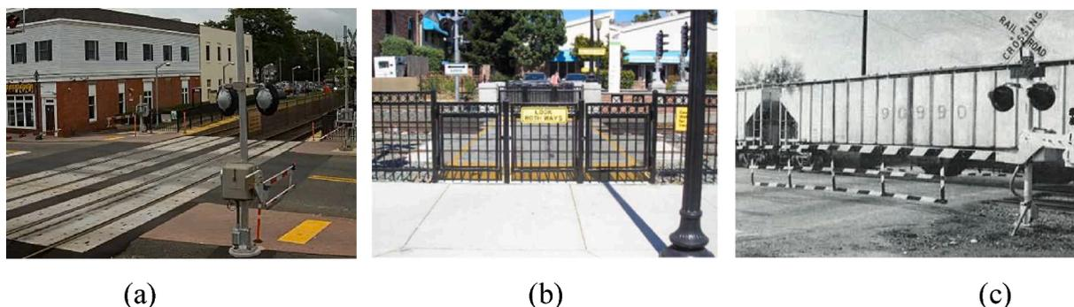
Fig. 15. Gate Options (a) Prototype Gate at the Selected Location; (b) Swing Gate in California; and (c) Gate Arm and Skirt at Knoxville, TN. Notes: Images: (b) California Public Utilities Commission, Pedestrian-Rail Crossings in California (c) Chase et al., 2013.
