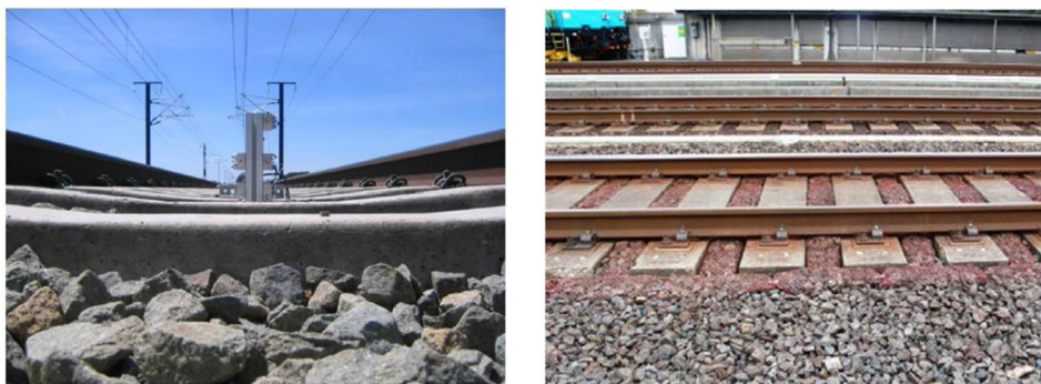
a) Ballast profile lowered on the Rome-Naples HSR b) Ballast Bagging, the solution proposed in Shinkansen, Japan
