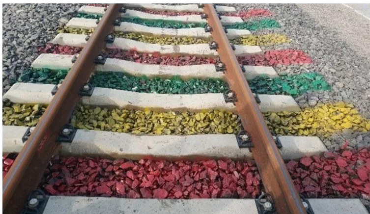
Fig. 14. Polyurethane ballasted track in the Ji-Qing line [72].
